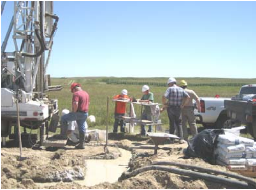
Well drilling in Logan County
