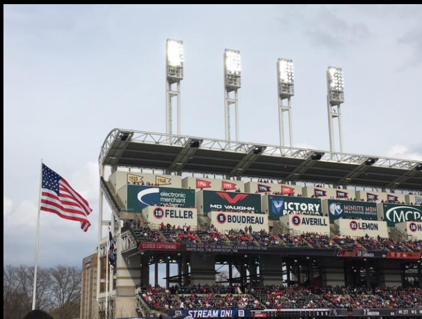
New lighting at Progressive Field Home of the Cleveland Indians
