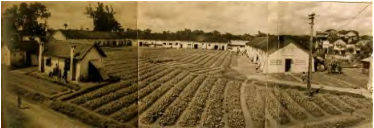
Central section of the Triều Khúc co-op facilities, 1948
