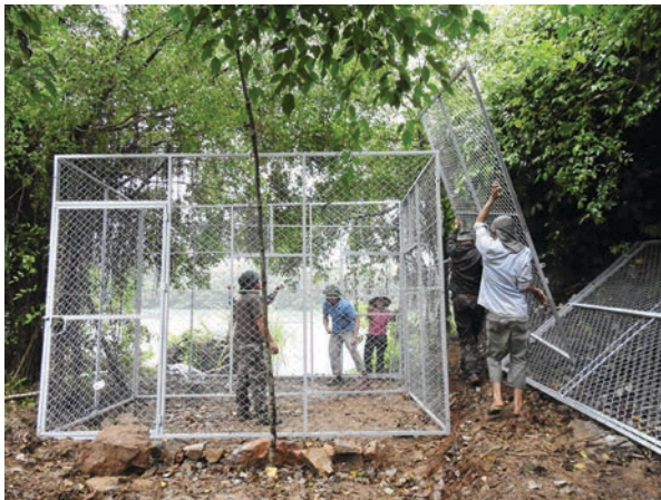
Fig.5. Erecting the cage on the island. Photo: Tilo Nadler.
