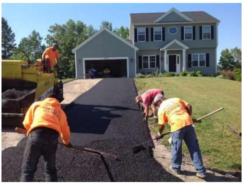
The best time to seal is 12 months after it has been paved, and every 2-3 years thereafter. Because blacktop is naturally porous, water can seep into and through paving. This not only causes deterioration, but results in ridges and upheaval due to frost and freezing. Blacktop is also softened and broken up by gasoline, lube oil, grease, road salts and anti-freeze which drips from cars. Sealer protects blacktop with a coating that is impervious to these harmful elements.
