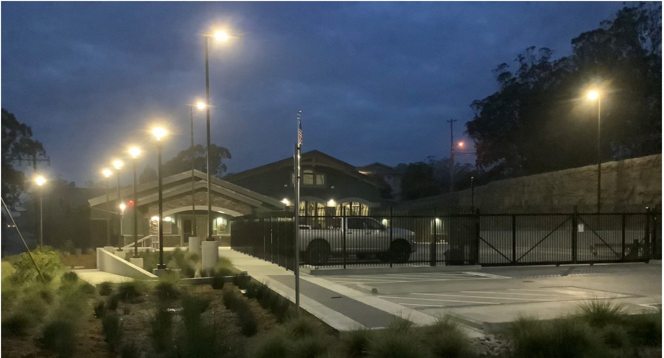
Photo 2: Post-construction lighting on the southeast side of the new fire station 41 with 10 light poles, 2 floodlights, sconces and base lighting at the flagpole.
