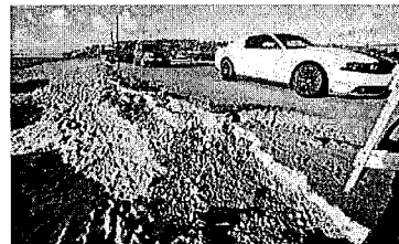
The heavy waves last year also cut into the side of Highway 101, eroding the shoulder.
