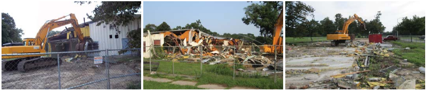
Building 56 (Community Store) – Demolition Activities
