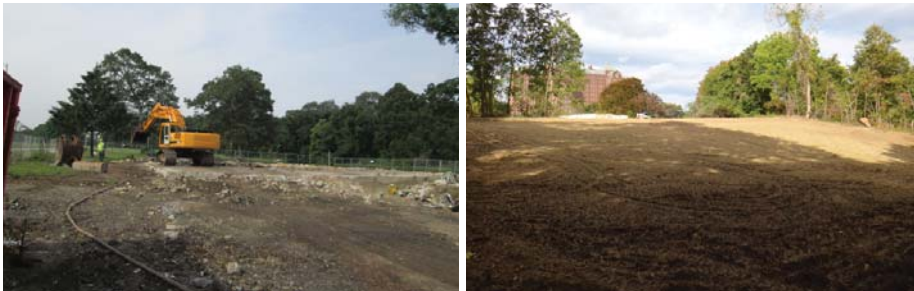
Building 82 (Morgue) – Site Restoration Activities
