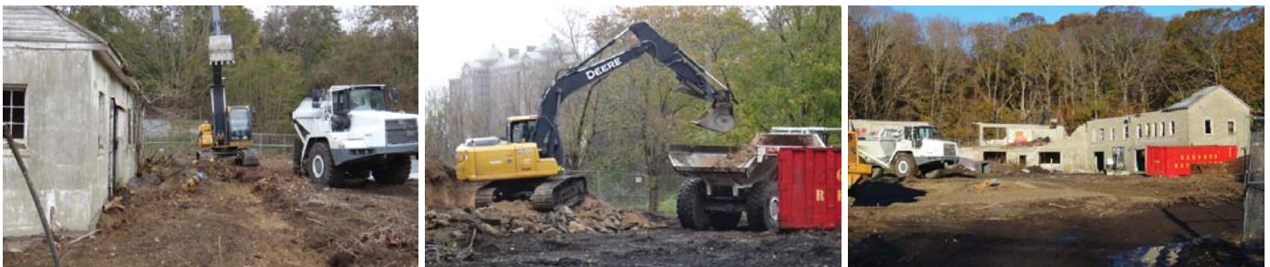
Building 47 (Dairy Barn) & 48 (Maintenance & Grounds) – Demolition Activities
