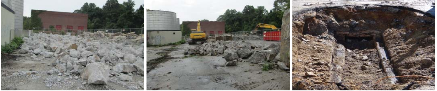
Building 56 (Community Store) – Site Restoration Activities
