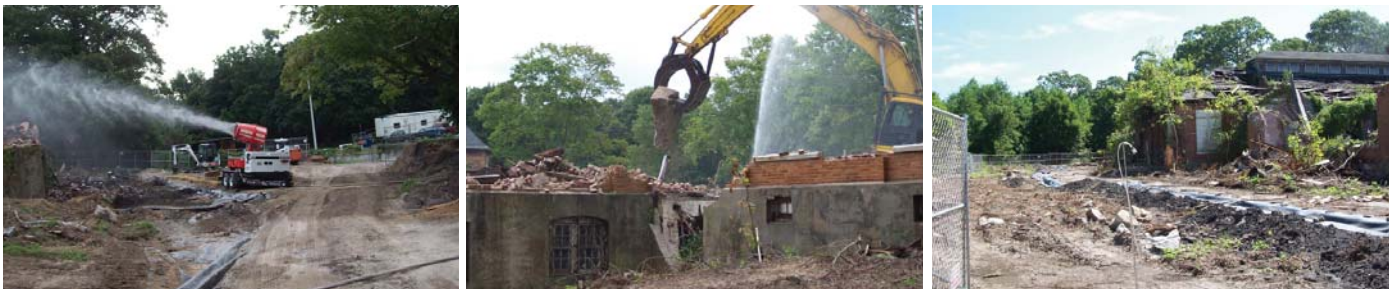
Building 122 (Inpatient 51 & 52) and Building 123 (Kitchen and Dining Room) – Controlled Demolition Activities
