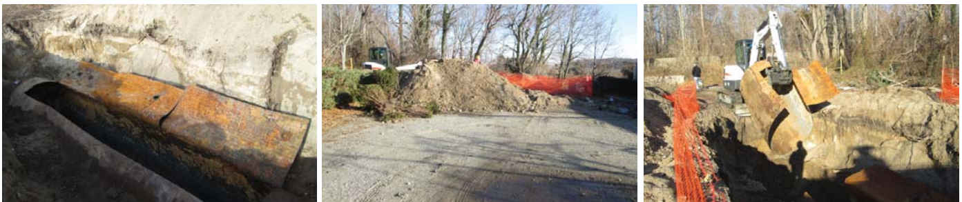
Barge – Demolition Activities (Site Work Only)
