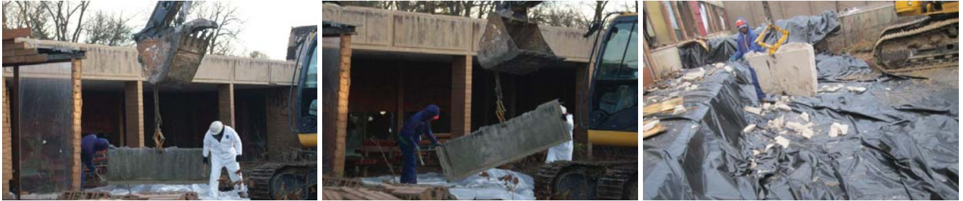
Building 23 (Buckman Day Treatment) - Demolition Activities
