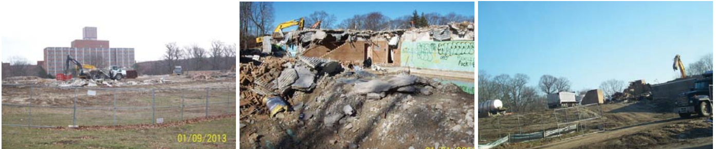
Building 23 (Buckman Day Treatment) - Demolition Activities
