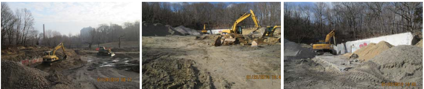
Building 47 (Dairy Barn) and Building 48 (Maintenance & Grounds) – Demolition Activities
