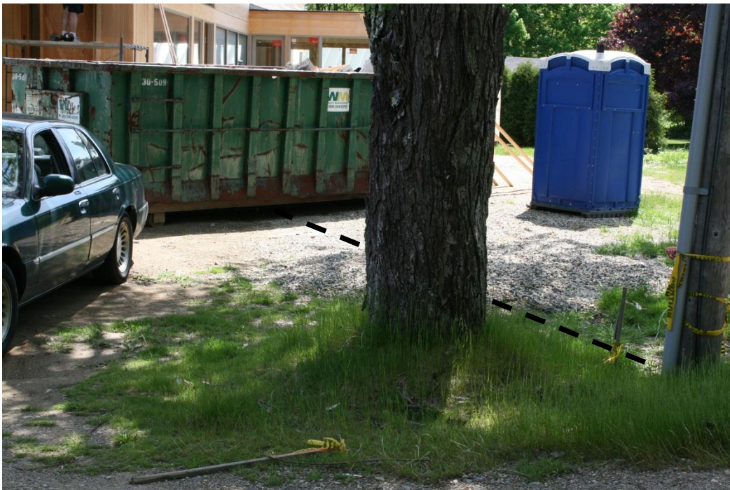
As no tree protection zone was established, the roots have been severely impacted by construction. The line indicates direction of utility trench.
