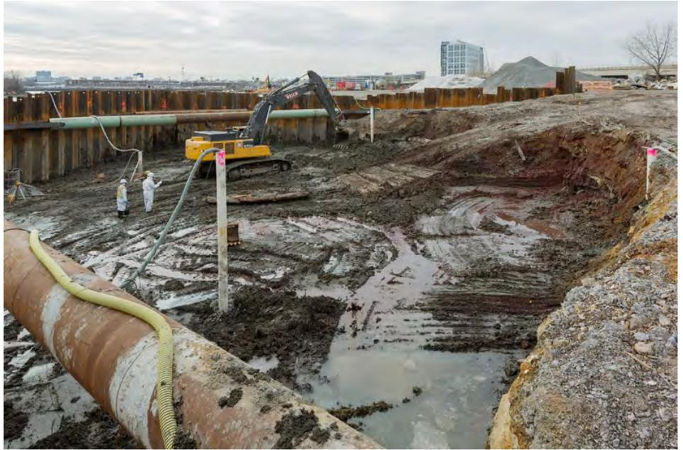
**To excavate the deeper layers of contaminated soil in Areas 1 and 2 groundwater had to be removed. Four wells in Area 2 were dug so groundwater could be pumped from the site.**
