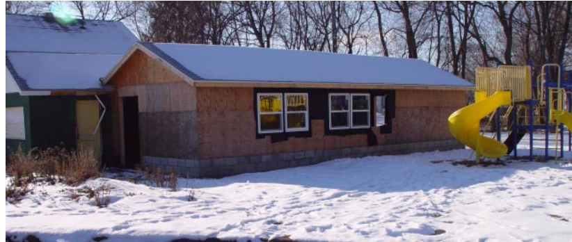
Figure 1: Community Center (under construction)
