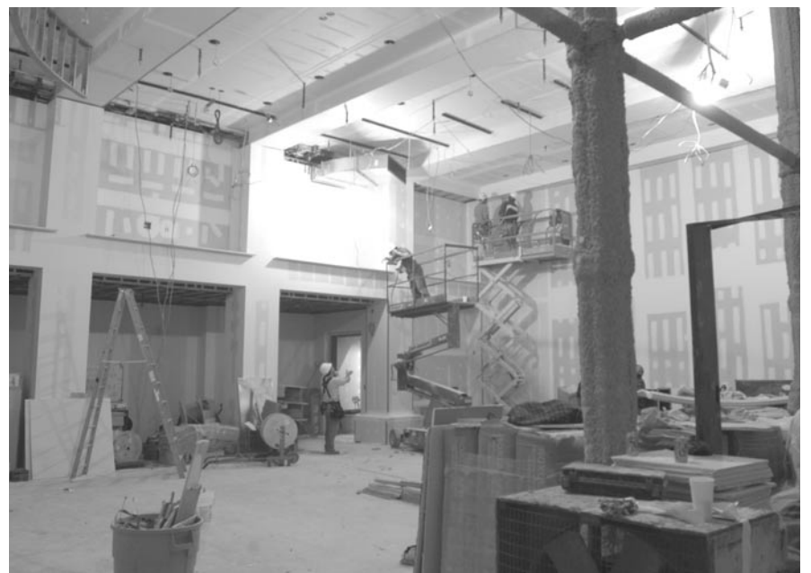
Work on East Hall, where the moonshine was found, nears completion.
