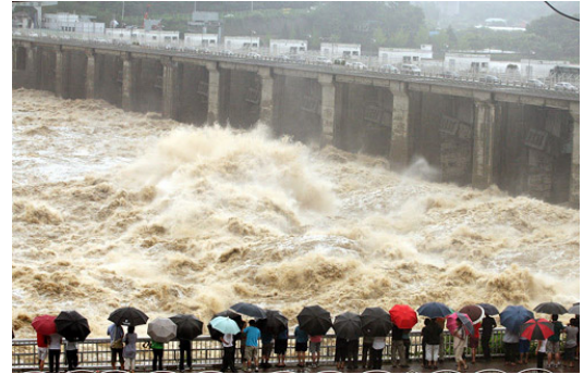
CHOSUN ILBO Paldang Dam, north of Seoul, 13 July 2009
