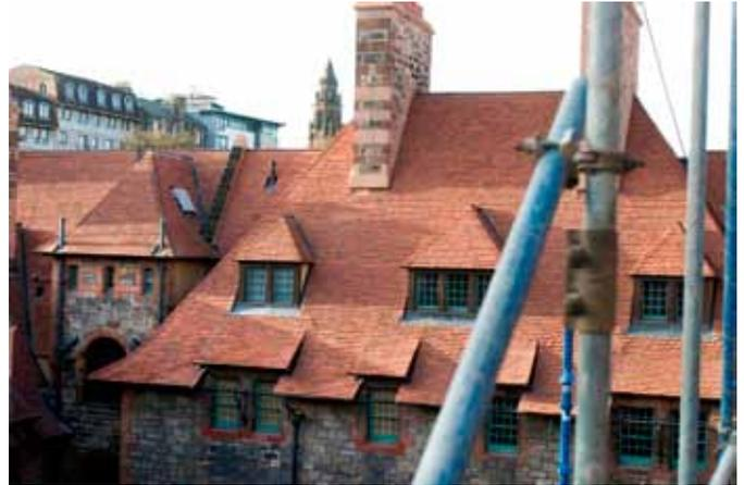
Chimneys have been re-built in Corsehill sandstone, carefully selected to match the original stonework. New decorative iron railings have been installed and stonework to the boundary walls is under repair
