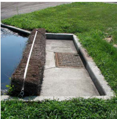
Temporary Filtration Device at Inlet
