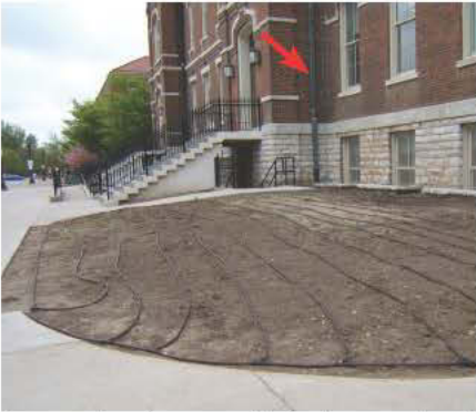
Irrigation lines being installed with external roof leader (red arrow) in the background. Perfect location for a cistern.
