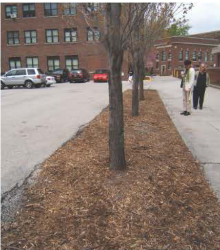
Curb-less, continuous, tree pit in campus core parking lot. Could be design for more storage capacity if grading allows.
