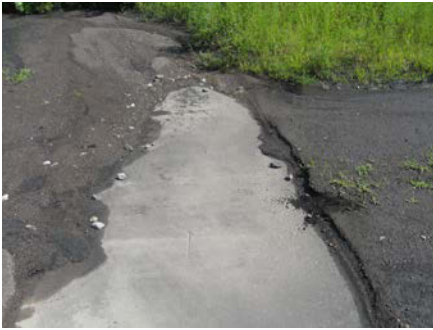
Accumulation of Particulate Matter on Concrete Slab where water is diverted to Harrison Pond.
