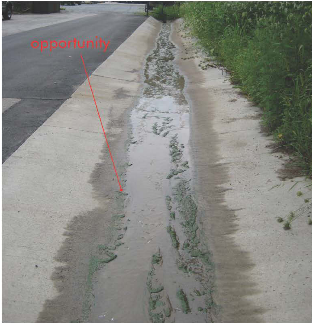
Equipment wash-down trough at golf maintenance area.
