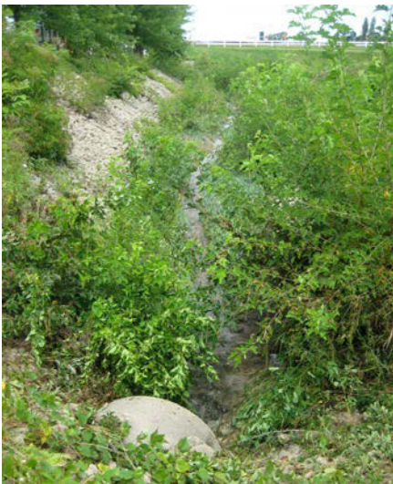
Shotcrete Stabilization Of Stream Bank - Cherry Lane In The Distance
