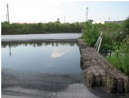
Temporary Filtration Structure for Surface Runoff along Service Road
