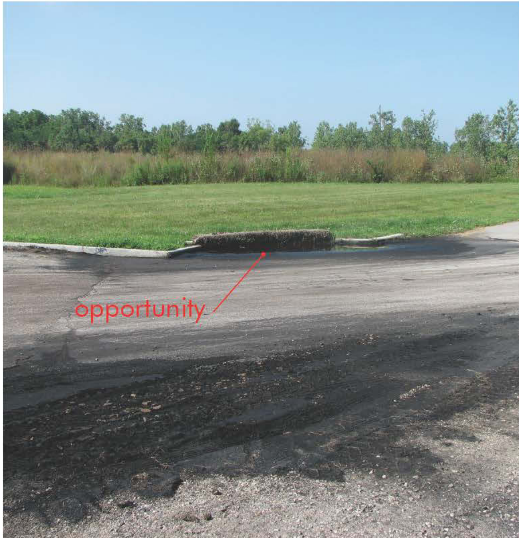
Inlet with Temporary Filtration Device in the Mid-ground, and Meadow in the Background.
