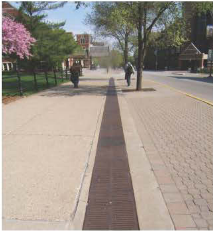
Trench drain in sidewalk next to Grant Street, by Purdue Memorial Union. Could be incorporated into a sub-surface continuous tree trench with hardscape on top.
