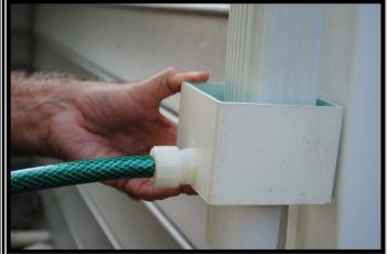
Step 8 - Fit the diverter to the top portion of the downspout.
