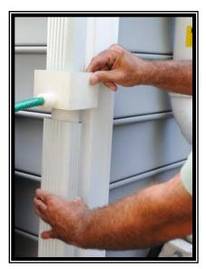
Step 9 – Connect the bottom portion of the downspout to the diverter.
