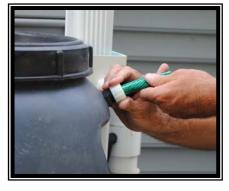
Step 12 -Connect the diverter to the rain barrel.
