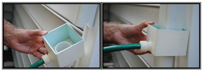
Step 8 - Fit the diverter to the top portion of the downspout. Below the top portion of the downspout (the part that is still connected to the house), orient your diverter so that the hose points towards where the rain barrel will be installed. Fit the diverter into the downspout. The downspout should fit snugly over the round PVC pipe in the diverter.
