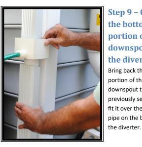
**Step 9 – Connect** the bottom portion of the downspout to the diverter. Bring back the bottom portion of the downspout that you had previously set aside, and fit it over the round PVC pipe on the bottom of
