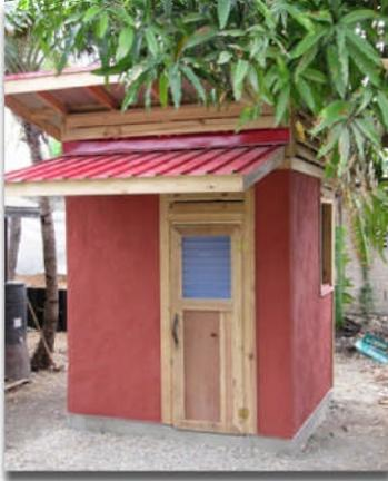
The **Senp Kay** introduced by Andy Mueller of GreenSpace Collaborative is the first structure in Haiti constructed utilizing prefabricated, tilt-up, plastic bottle filled panels and light straw-clay walls. It was designed and constructed as an innovative solution for low-tech, sustainable housing for low income communities in emergent nations.
