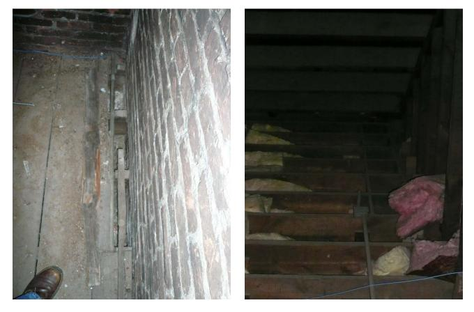
A contractor with a specialty in air sealing, not just insulation, should be hired to air seal all areas first. Once the air sealing has been completed the entire attic should be insulated with blown insulation to a minimum total R-value of 38. This additional insulation can be installed directly over the existing fiberglass batts.
