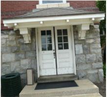
Many of the exterior doors do not seal well and are therefore leaky. Make sure weatherstripping is installed on all exterior doors and that it is in good condition. Small cracks add up and can have a large impact on heating and cooling energy.
