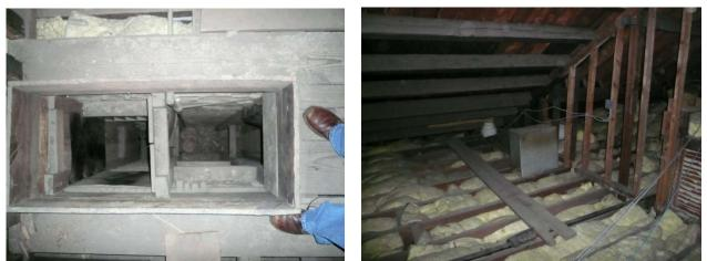
series of ventilation shafts tied to ductwork in the attic. The system worked via natural convection with hot air rising up through the building and being ventilated through vents in the roof and gable ends of the building.
