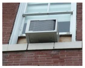
HVAC system at the Mellor Building is its inability to provide outside air to occupants. Outside air still enters the building through open or leaky windows, but this uncontrolled method of infiltration is certainly not preferred from an energy standpoint. The following HVAC recommendations consider the pros and cons of a number of potential replacement systems or retrofits which intend to improve the energy, comfort, acoustic and aesthetic performance of the current system.
