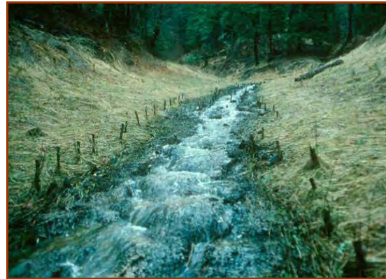
The soil-filled TRM (Enka Mat) protected the channel immediately. Reinforced with live staking. (J. McCullah, 1992)
