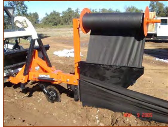
Silt fence installed by slicing method.
