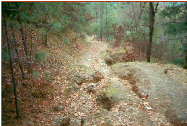
The gully causing runoff on this road/trail can be dispersed by outslowing the trail.
