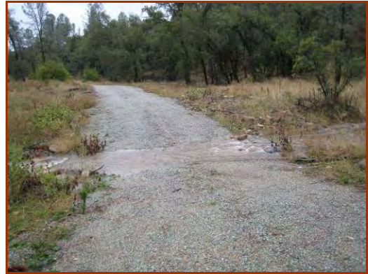
This ford or “armored dip” has a well-compacted structural sub-base (large cobbles) and then armored with stone. (J. McCullah photo, 2007)
