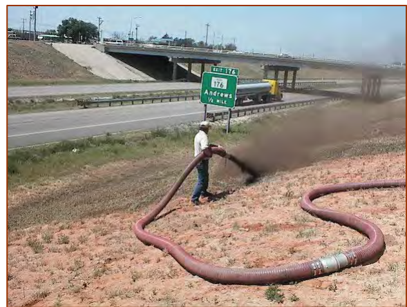
A 2 inch thick compost blanket, applied pneumatically for surface stabilization. (Photo Courtesy of Texas DOT.)
