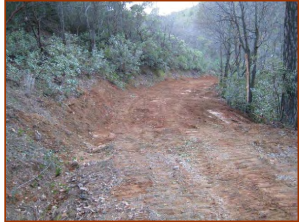
On this same road, just before the transition from inslope to outslope, a rolling dip is constructed to take runoff from the inslope section off the road.
