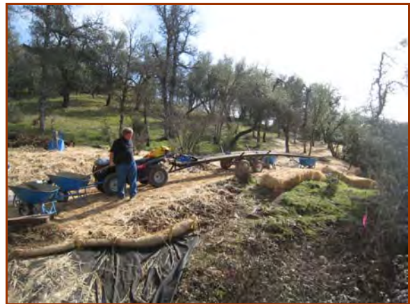
Fiber rolls can be used to protect stream crossings when developing new trails. (Gold Run Creek Trail, Redding, CA)
