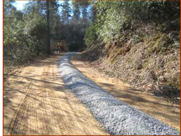
20T of base rock dumped in a downhill direction with a “bellydump” is ready for spreading.
