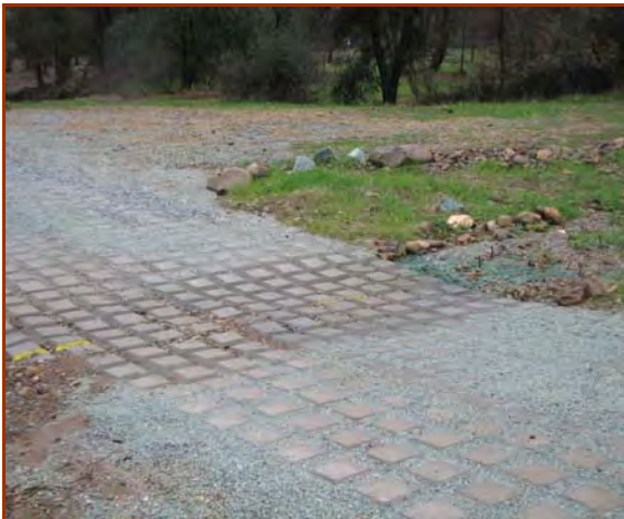
A cabled ACB after one year and several big storm flows in a watershed restoration project.
