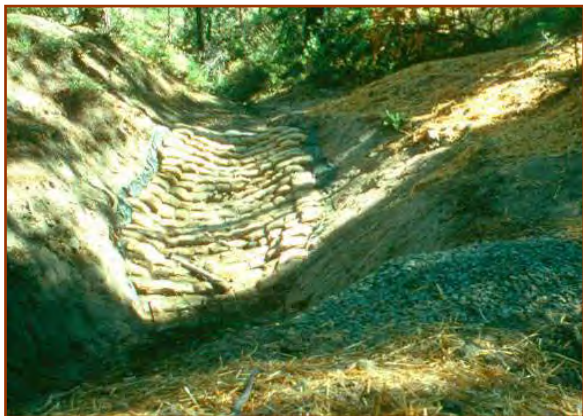
Headcut structure made from soil/cement sandbags structures.
