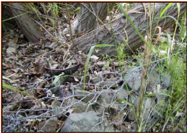
This rock-filled gabion has a 10 year-old willow tree growing through it with no deformation or “lifting”. There is ample proof that woody vegetation will only reinforce gabions, not cause structural compromise.
