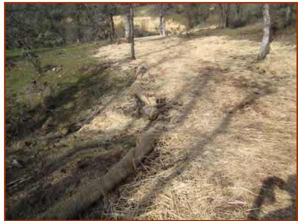
This outsloped recreational trail was designed with rolling dips and terrain dips. (Gold Run Creek Trail, Redding, CA)
