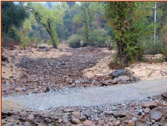
This ACB system is in-filled with ¼ inch granular aggregate to help lock blocks together.
