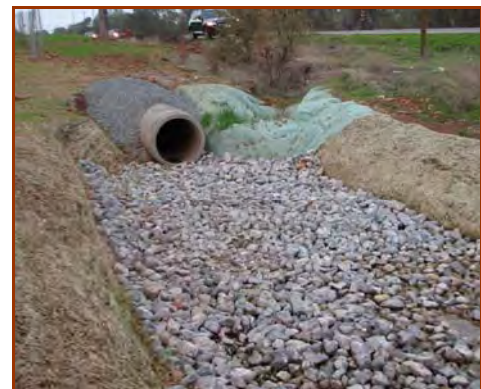
Riprap apron-type Energy Dissipator.
