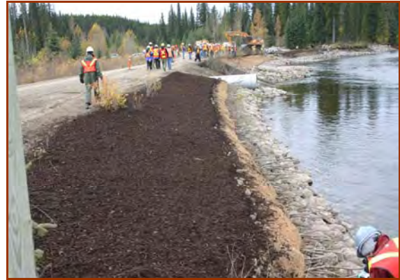
Compost blanket at vanes 2 and 3. Note that willow cuttings were also incorporated into this streambank protection design. (2005)
