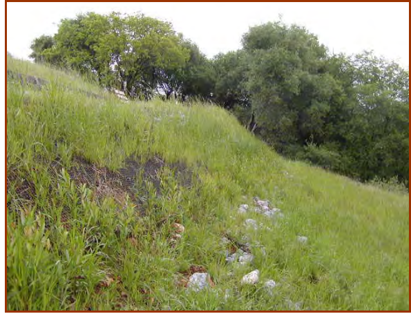
SS-3 Mycorrhizae Inoculation aided in vegetation establishment for adverse soils on the Old Hwy 99 Road to Trail Project. The photo on right shows the Vegetated MRE after 5 months (Redding, CA, May 2003).
