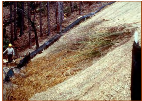
Live Gully Fill Repair relies on the use of willow branches (and sometimes geotextiles) to provide soil reinforcement. (J. McCullah photo, 1994)
