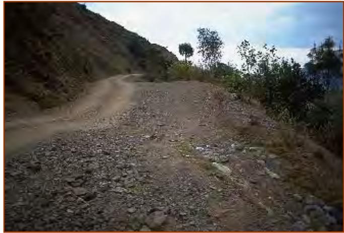
Low gradient roads with a competent rock surface can achieve sheet flow drainage with a 2% outslope.
