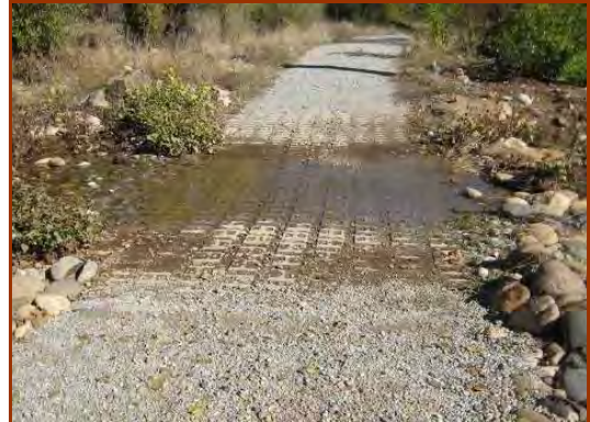
This low water crossing, designed for recreation and heavy equipment, is constructed from Articulated Concrete Blocks (ACBs). (J. McCullah photo, 2007)
