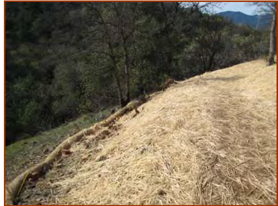
The "stake and rope method" of anchoring fiber rolls was used for sediment control along this outsloped recreational trail.
