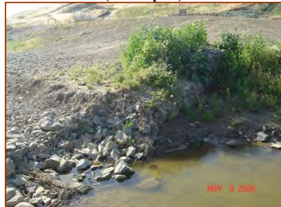
Gabion wire is abraded by stream sediment and corroded by water until the structures fail. (J. McCullah photos)
