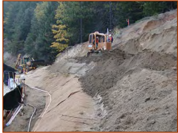
The adverse soil on this decomposed granite slope was stabilized by using a 25% compost mix.
