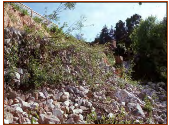
Vegetated gabions after only 4 months (Branciforte Creek in Santa Cruz County). The willow poles were inserted through the baskets during construction, then backfilled with rock. (J. McCullah photos)
