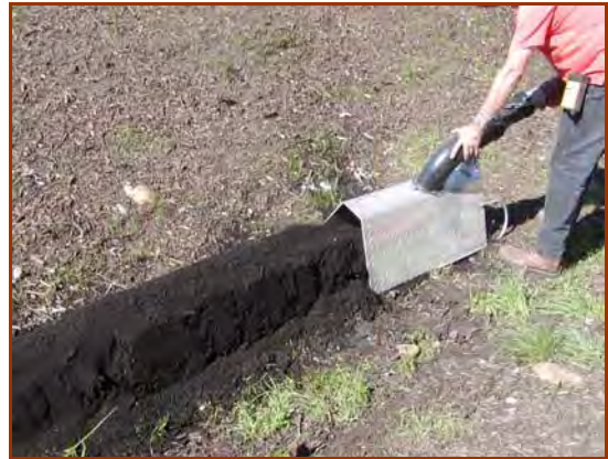
Compost berms are relatively new Best Management Practice (BMP) sediment control technology.
