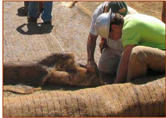
A coir composite TRM being installed and anchored into a check slot.
