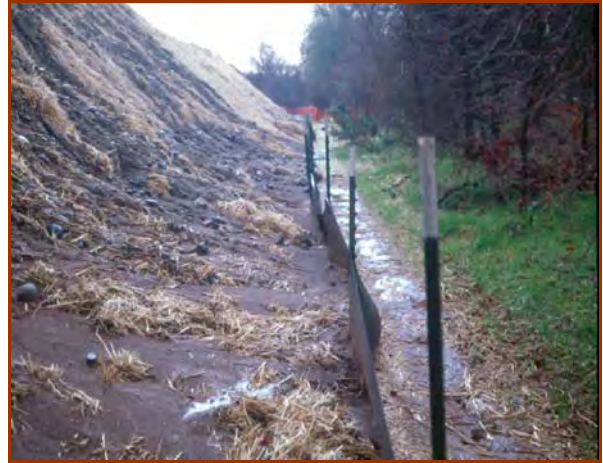
This huge stockpile was stabilized through the winter with straw mulch and silt fence installed by "slicing" with a silt fence machine (see PO-5 Stockpile Management).
