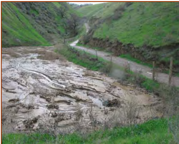
Sediment ponds need to be cleaned out prior to the rainy season, and the sediment needs to be stockpiled and properly protected.
