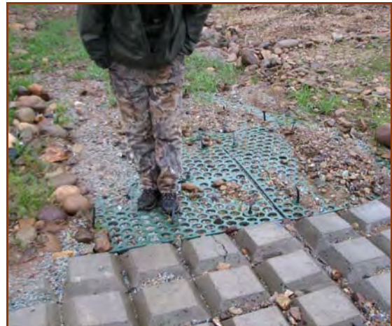
Scour Stop® can be vegetated. Here it is used for outlet transition and channel protection. (J. McCullah photos, 2006)
