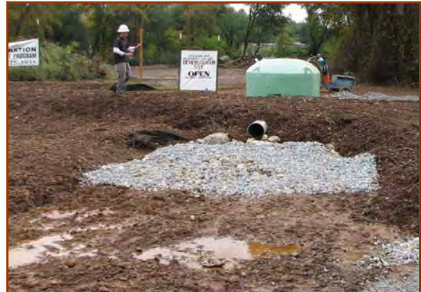
Apron is "overcut" to accommodate riprap thickness, and then lined with anchored geotextile.
