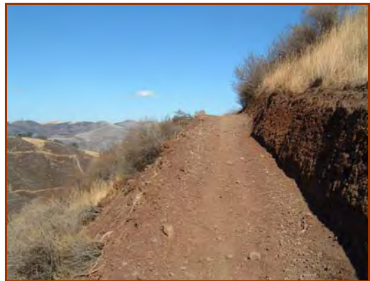
Construction of new SVRA trails should cause minimal disturbance by following natural land contours. (Carnegie SVRA)
