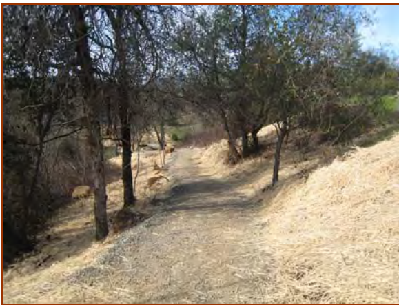
This outsloped recreational trail was designed with rolling dips and terrain dips. (Gold Run Creek Trail, Redding, CA)
