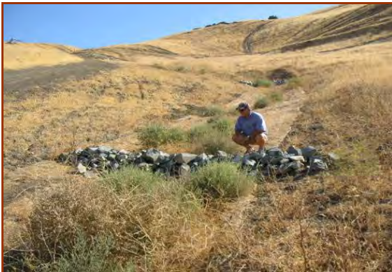
This rock check dam needs a lower weir crest to avoid "end runs".
