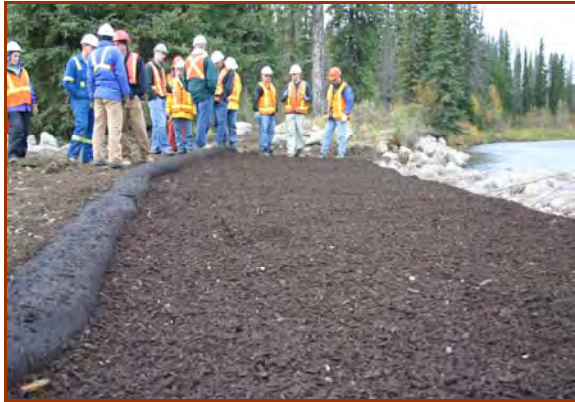
Two-inch thick compost blanket installed on Alberta DOT streambank project (at vane 1). Note compost sock installed for sediment control. (Canadian Rockies 2005)
