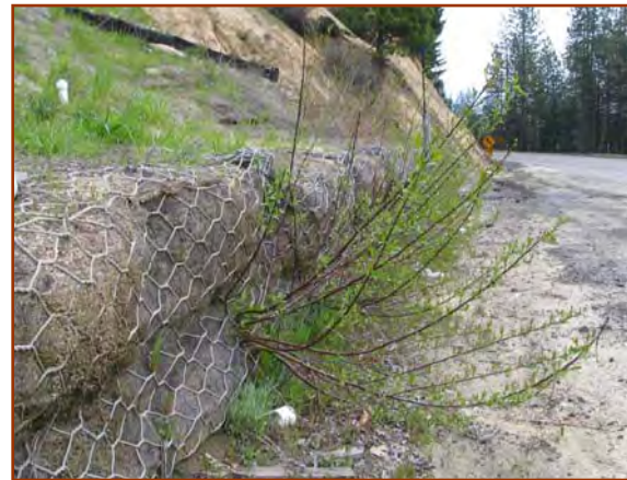
Vegetated (willow pole) gabions at the toe of a highway cutslope in Trinity Hwy 299W. The deeply planted willow pole plantings are at 3000' elevation and have survived four summer seasons (100° F plus).
