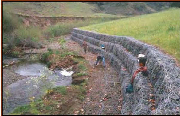
Morrow Creek, Morrow Bay, CA (March 1999). Scour apron being planted with Live Staking “after the fact”. It is very difficult to plant gabions after construction.
