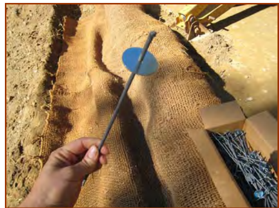
Metal stake pins with steel washers may be used for anchoring ECBs.
