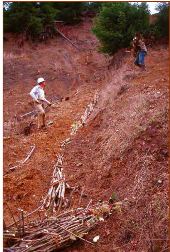
The gullies were packed with Live Pole Drains (Live Fascines) to allow subsurface drainage.
