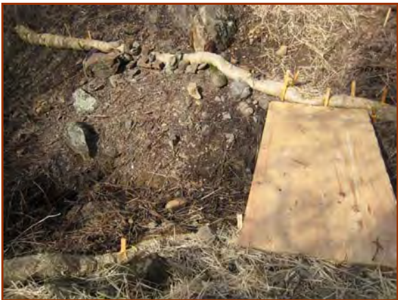
Fiber rolls can be used to protect stream crossings when developing new trails. (Gold Run Creek Trail, Redding, CA)
