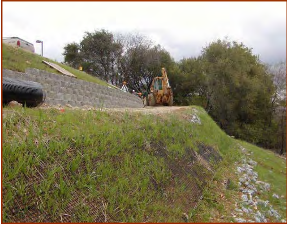
SS-3 Mycorrhizae Inoculation aided in vegetation establishment for adverse soils on the Old Hwy 99 Road to Trail Project. The photo on right shows the Vegetated MRE after 5 months (Redding, CA, May 2003).
