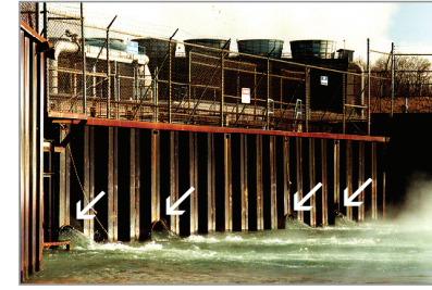
Water discharge area at the Palisades nuclear power plant on Lake Michigan. Note the flow from four big ejection outlets .
