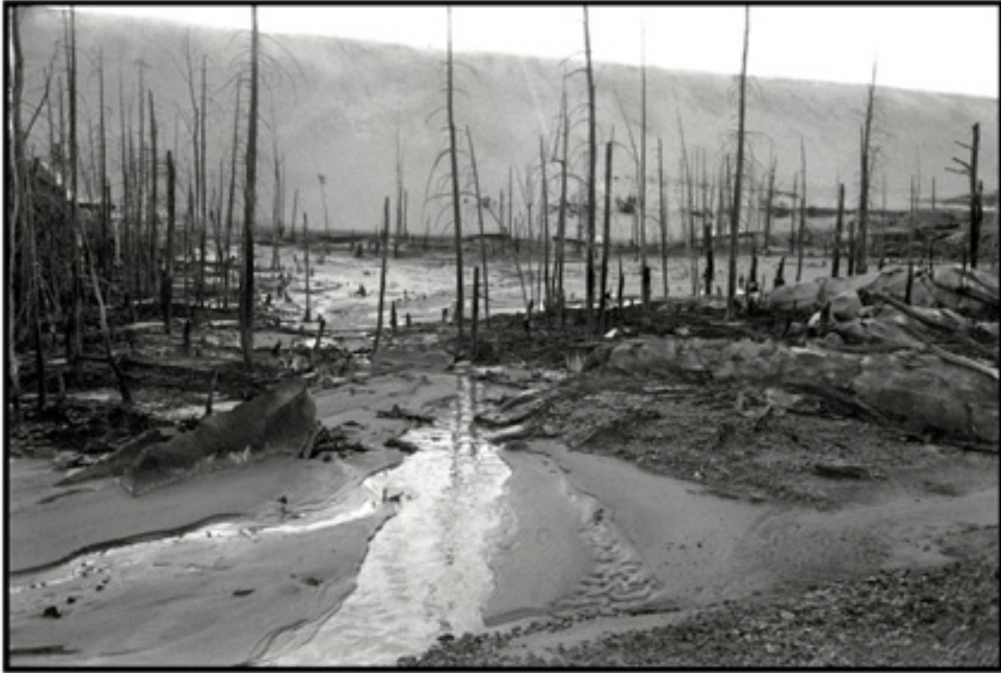
Stanrock Mill Tailings Area, Elliot Lake, Ontario, 1986. The 30-foot high wall of white sand behind the trees is made up of uranium tailings. Over 130 million tons of these tailings have been deposited in the Elliot Lake region and have contaminated the entire 58-mile long Serpent River system, finding their way into Lake Huron. (Photo: Robert Del Tredici.)
