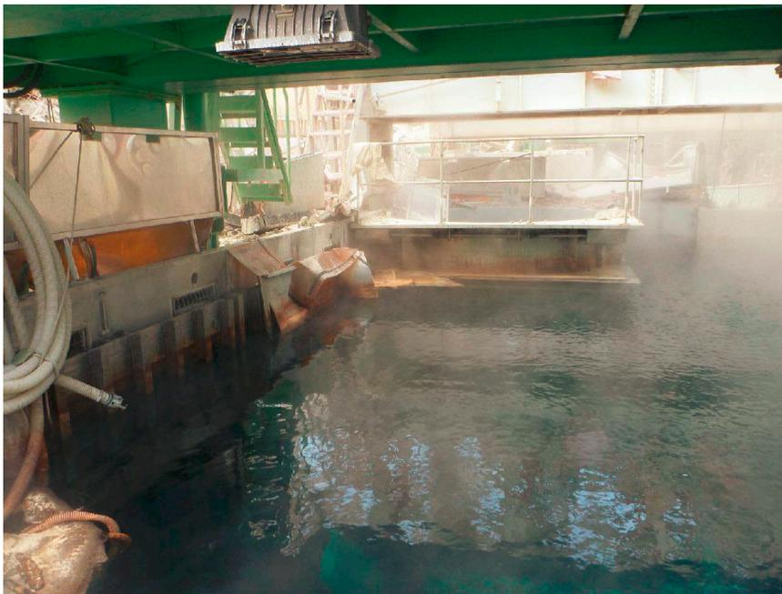
FIGURE 2B.2 Water evaporating from the surface of the Unit 4 spent fuel pool. SOURCE: TEPCO image released June 29, 2011.
