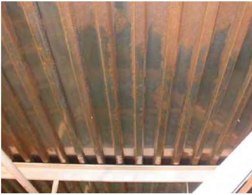
**Figure 12:** Corrosion of a Type 304 stainless steel roof deck above an indoor swimming pool.
