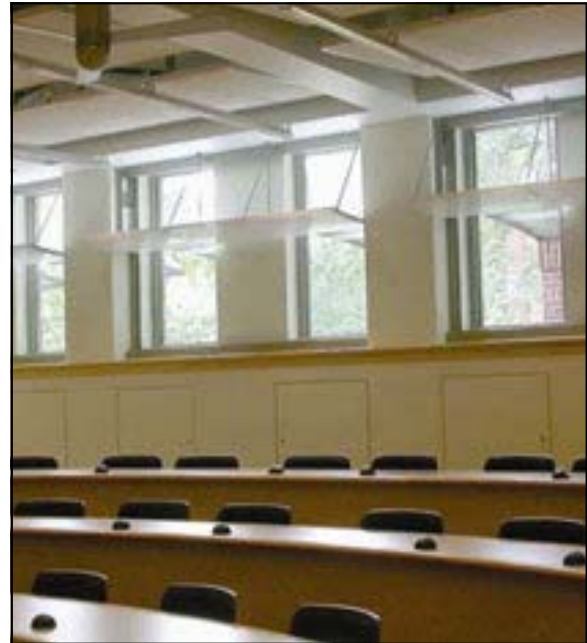
Lillis Business Complex with external shading devices and interior light shelves.
