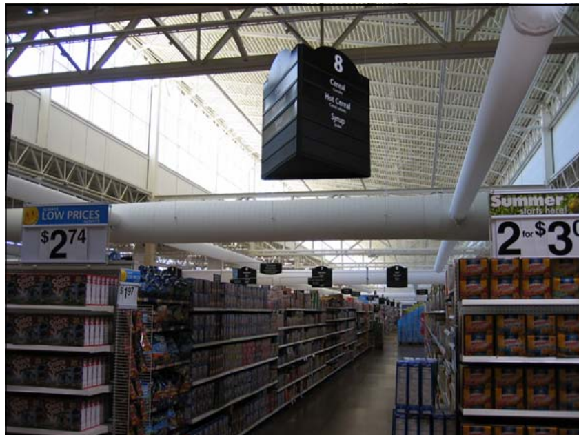
Diffuse top lighting throughout Walmart in Aurora, Colorado help reduce the need for electric lighting.
