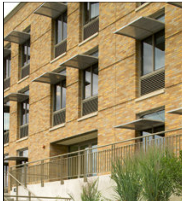
Mount Angle classrooms with external shading devices with interior light shelves.
