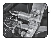
Mount the Flasher to the L-Bracket using the extra bolt threads from step 8 B. Use the thin, locking jam nut provided.
