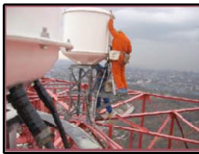
Job Site: TTI Tower Elevation: 990' Microwave Antenna Installation & DSI Staff Member
