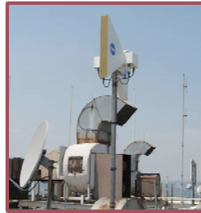
Job Site: Legg Mason Building Quad Antenna Installation
