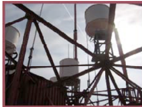
Job Site: TTI Tower Elevation: 990' Microwave Antenna Installation Completed
