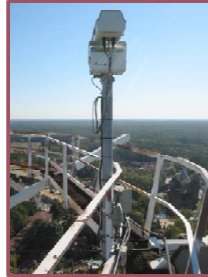
Job Site: Jackson, NJ Camera Installation atop Roller coaster
