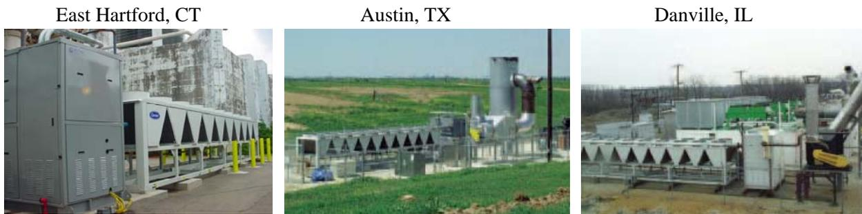
Figure 5. Existing HVAC-derived ORC installation
