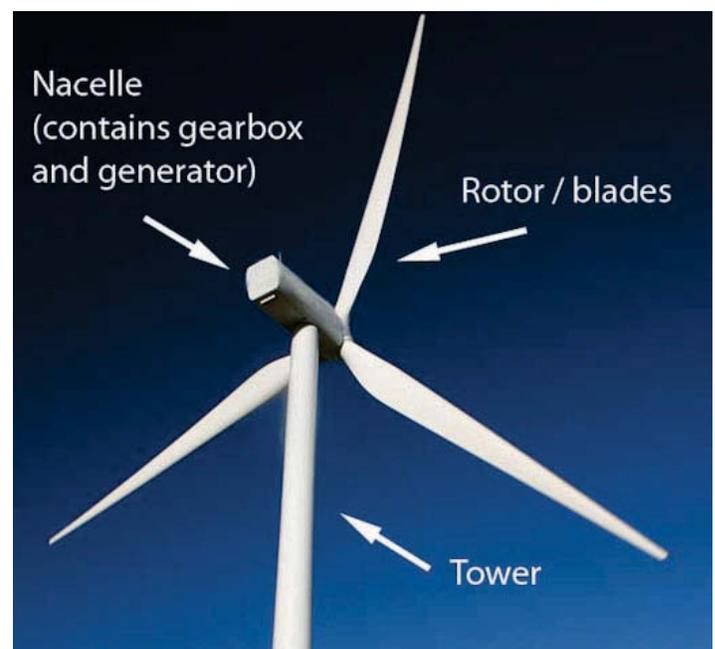
**Figure 3: Wind turbine components**
