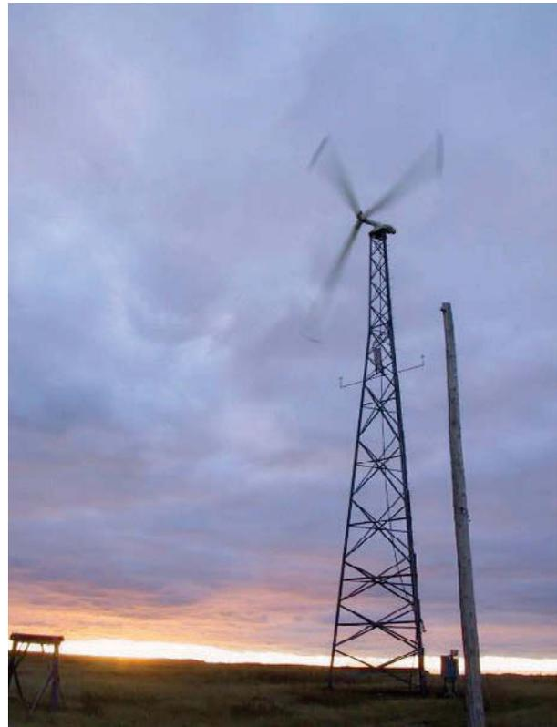
**Figure 5: Lattice towers are sometimes used for small to medium-sized wind turbines**
