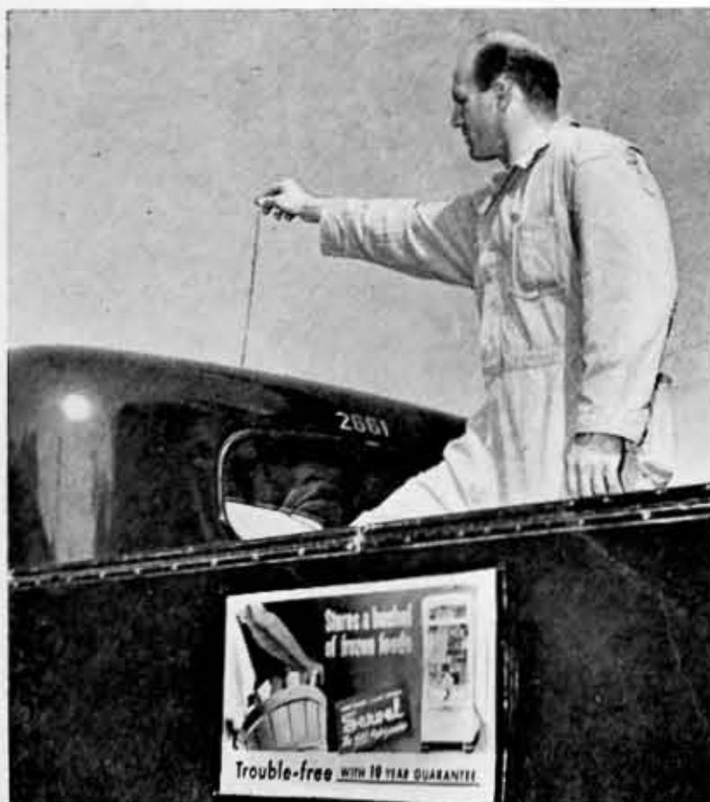
ANTENNA is placed on top of the cab. Three such units are now in operation in service cars in the Pasadena District and more will be installed in future.
