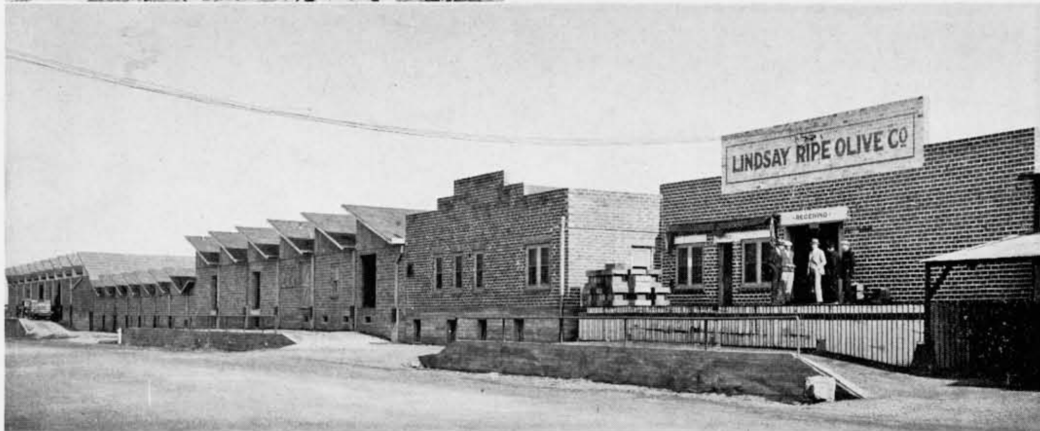
Above—Fig packing plant of Beckwith Company, Reedley. Below—Plant of Lindsay Ripe Olive Company, Lindsay, largest olive packing plant in the world.
