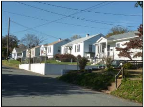
Housing for Ix Mill Workers
