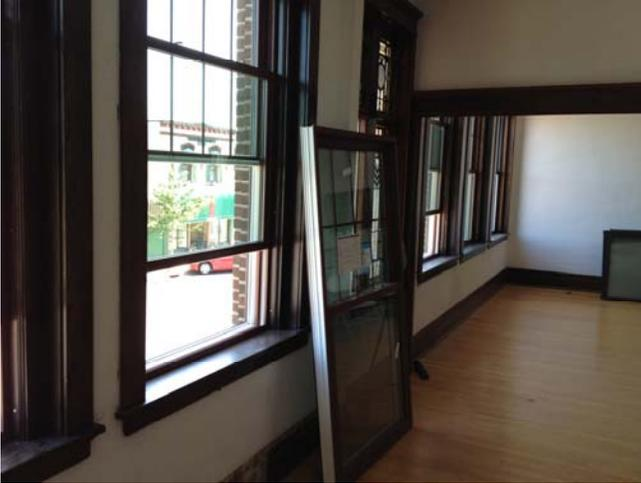
5 of the 6 Windows are installed in the Dining Room and Club Room. The Window in the foreground was damaged in shipment and is being replaced. Each of the windows that was replaced had rotted in the frames, some worse than others, and wood had to be replaced to install the windows. The installer stated that this was a larger job than originally anticipated. He is very good at what he does and I could tell he was very meticulous and skilled. He is doing an excellent job.
