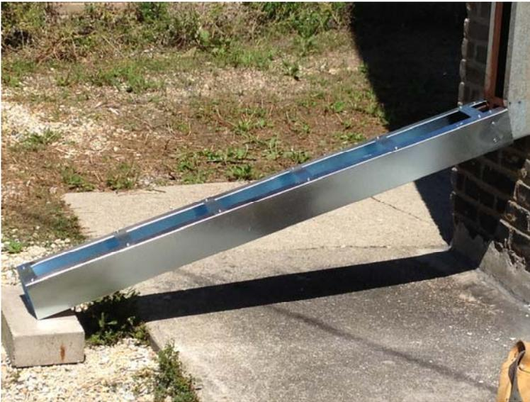
New custom fitted down spout extensions that match the original down spouts, diverting water away from the foundation of the building. You can also see in this photo and the bottom corner of the building that they have closed gaps, cracks and crevices that were letting water into the foundation. They used caulk and grout (for lack of the appropriate term).
