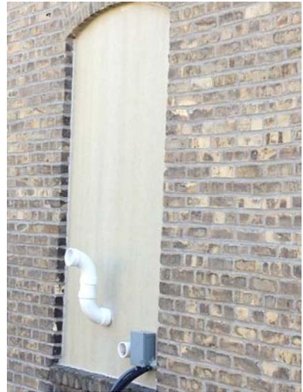
Photo of the Hardie Board replacement (fiber/cement) on the side of the building where the Barbershop AC Unit is located. Not Painted yet. Exhausts were re-done, lessening chance of Carbon Monoxide (CO) by appropriately venting out of the building. This replaced plywood, fiberglass insulation, newspapers and paper catalogs that were found during the removal and replacement with the Hardie Board.
