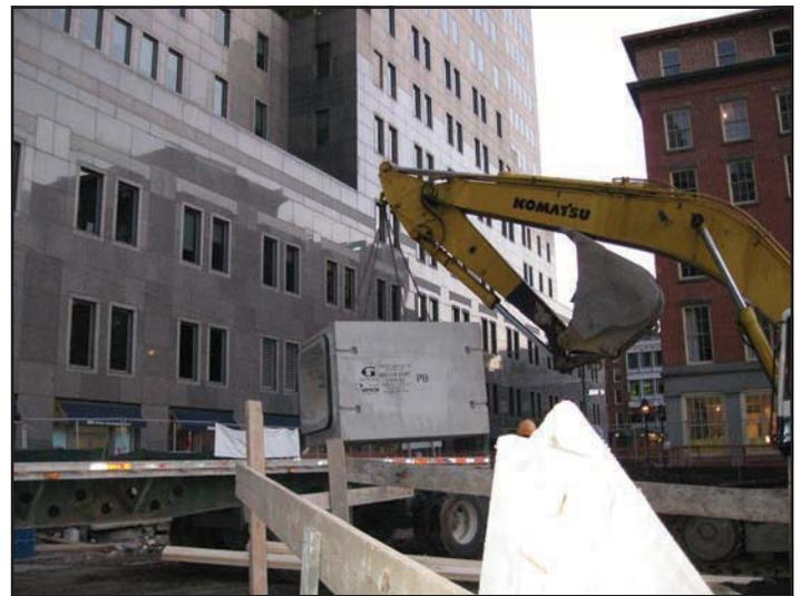
**A concrete box culvert is lowered into place.**
