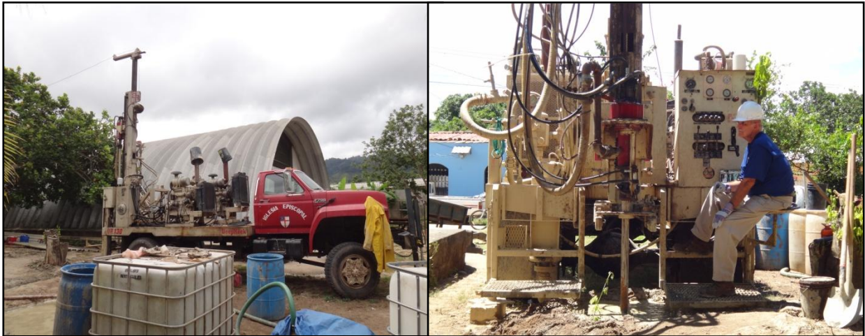
Drilling with our medium sized rig, the DR-130
