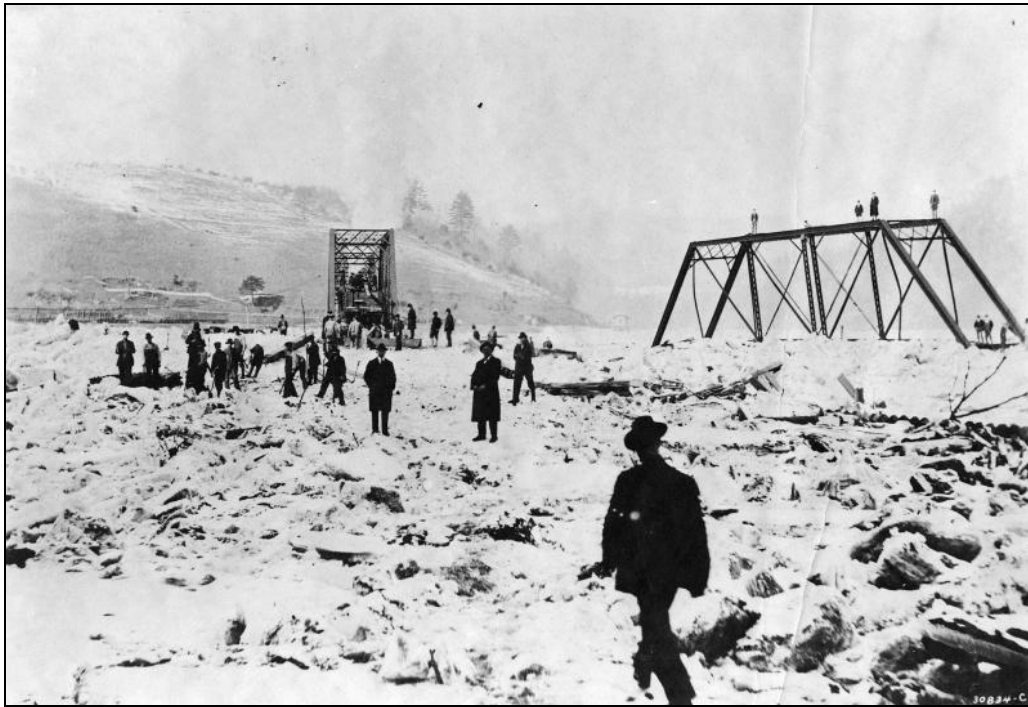
Figur 9 Damage of a steel bridge due to ice jam and flooding.
