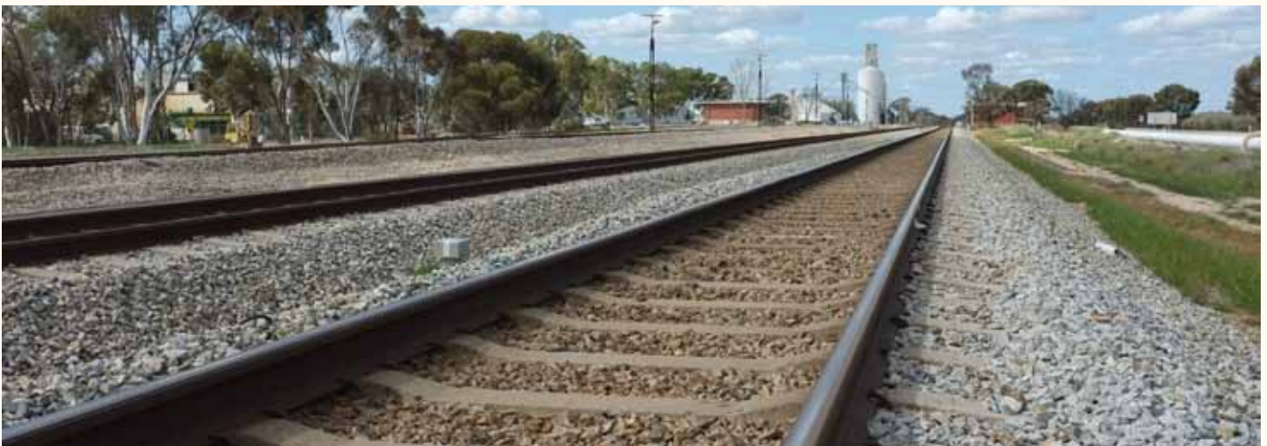
Rail line showing high levels of weed control. Photo: A Storrie
