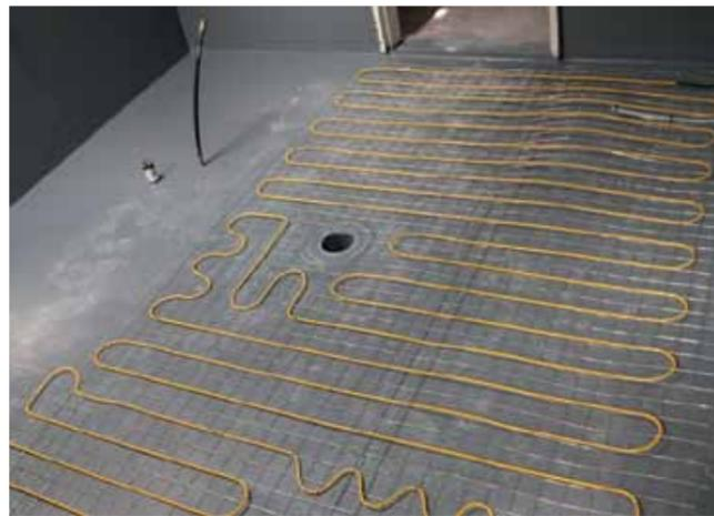
**Above** Bathroom screed installation is the most common bathroom installation used, placed directly over the waterproof membrane before the floor tiles are laid. "Only the free floor space is used and the cost is very affordable. Bathroom heating becomes totally invisible within the smallest room in the house," explains Sandra Skelly of Comfort Heat
