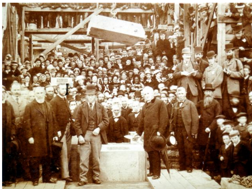
Laying the foundation stone of the new Free Church in Comrie, 24 September 1879. James Carment is on the left of the front row.
