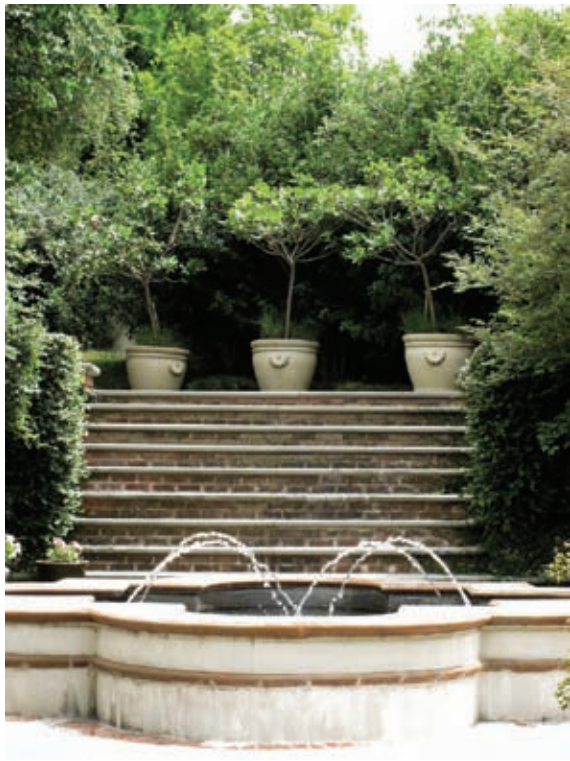
This quatrefoil shaped fountain is placed on a center-axis to the main garden and the house. The coping is acid stained concrete and is at a height to provide additional seating.
