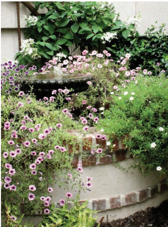
This small, secluded fountain was designed to be viewed from only one window. It's stucco with a brick cap and watertable with a cast iron basin. Lush plantings surround the fountain and provide a softening effect.
