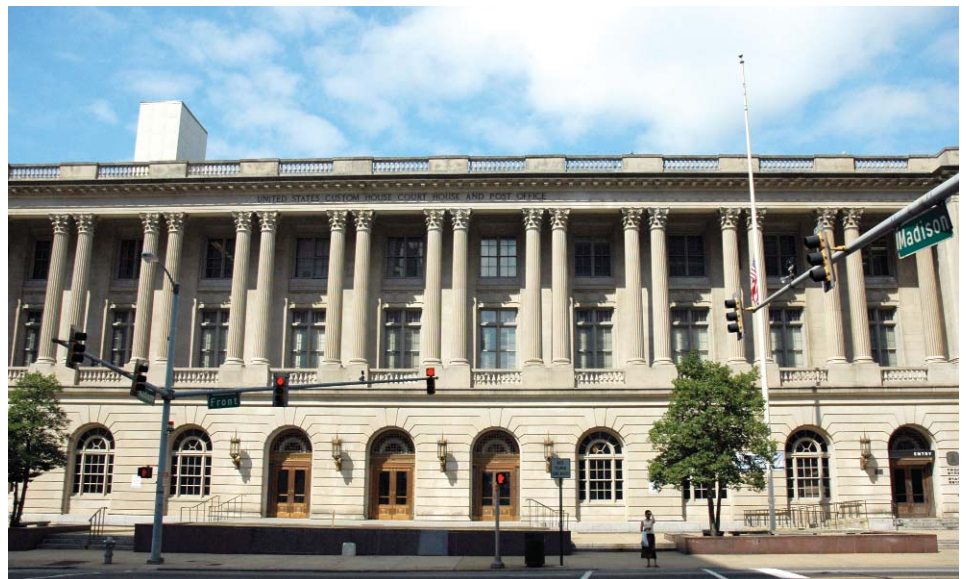
In August 2009, the Cecil C. Humphreys School of Law will move to the historic customs house, courthouse and post office — pictured above — in downtown Memphis.
