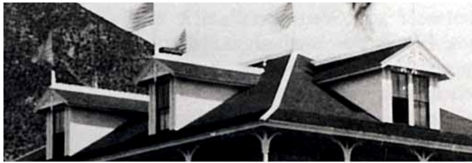
Figure 9: Dormer detail showing the Eastlake/Stick elements above the window
