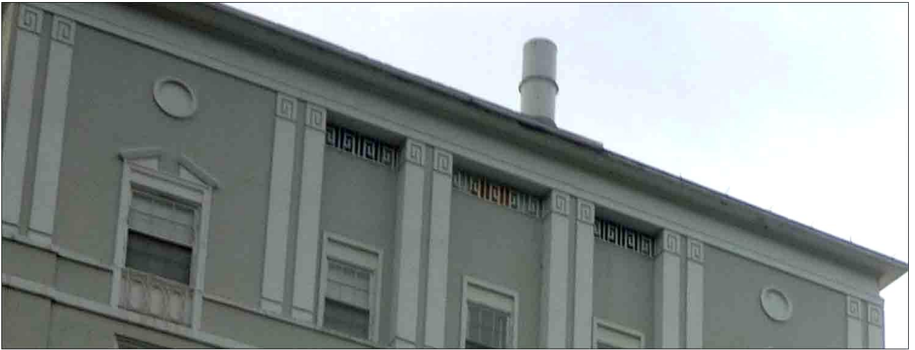
Figure 18: Pilasters with Capitals bearing a Greek Key design that is repeated as a fret pattern under the eave inset.
