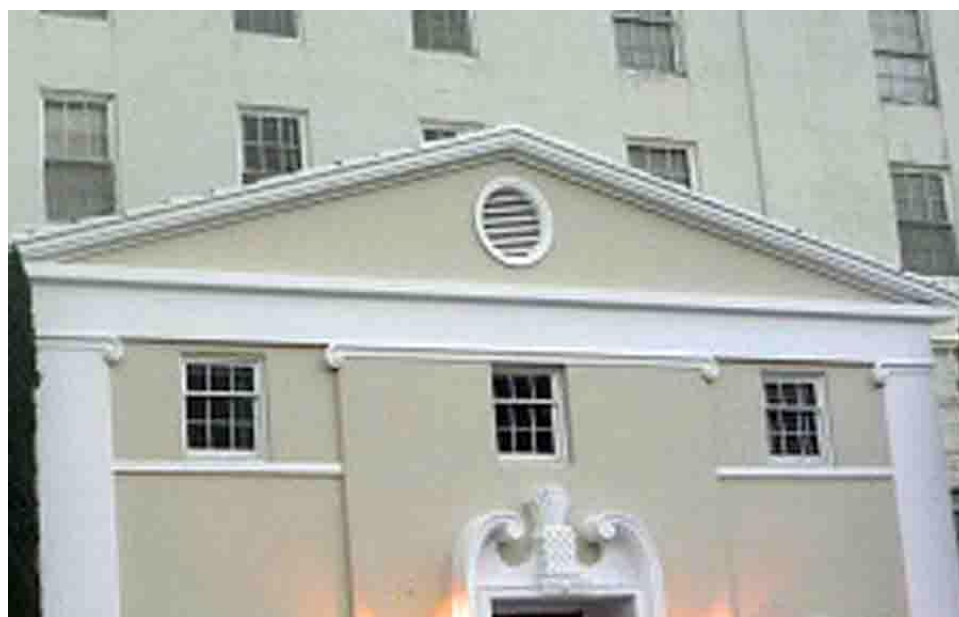
Figure 17: Compressed Greek Ionic capitals below the triangular pediment
