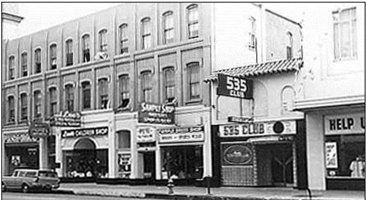
The Commercial Hotel, 525 W. Third Street
