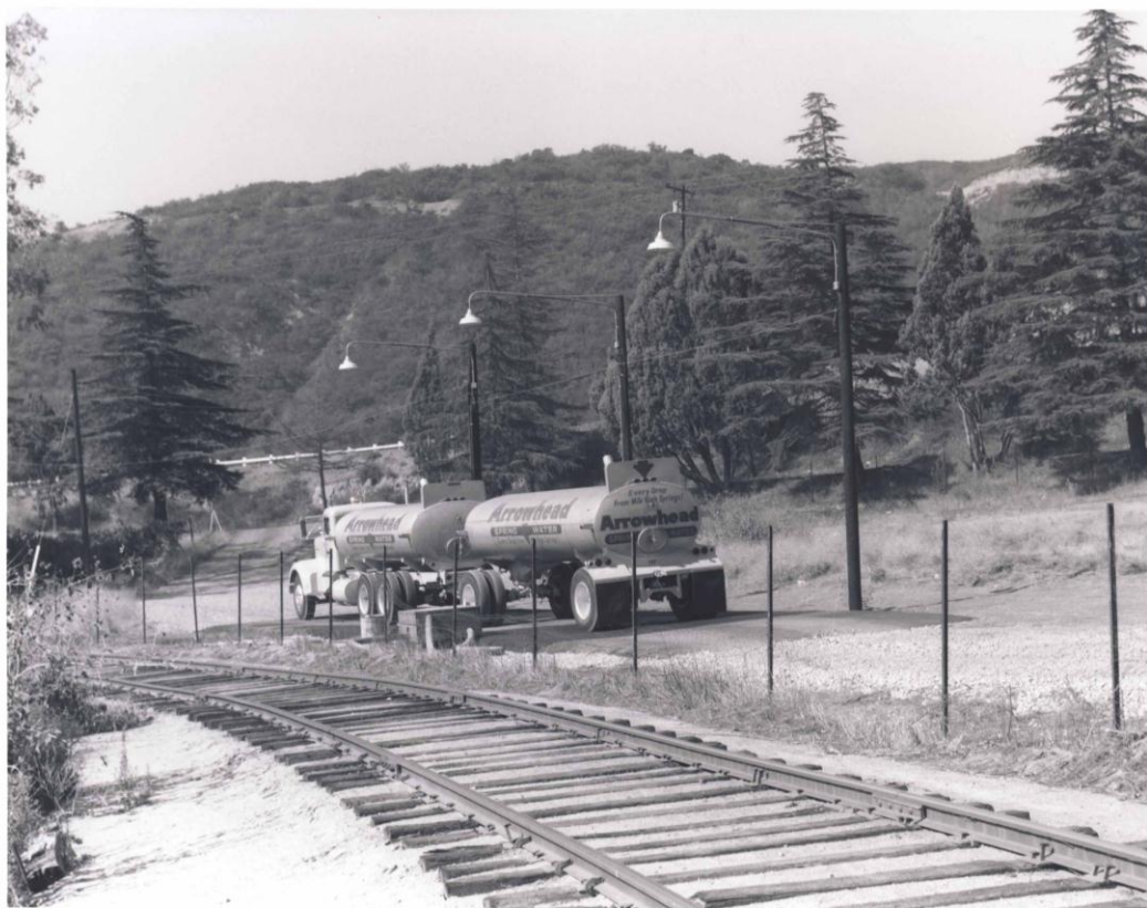
This photo, contributed by freelance correspondent Mark Landis, shows the entrance/exit for trucks to the loading rack, virtually using the same alignment as the old railway
