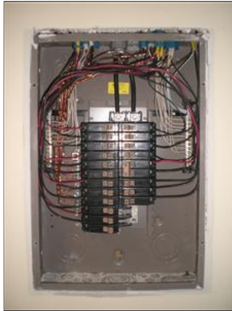
7.1 Picture 5 basement storage
