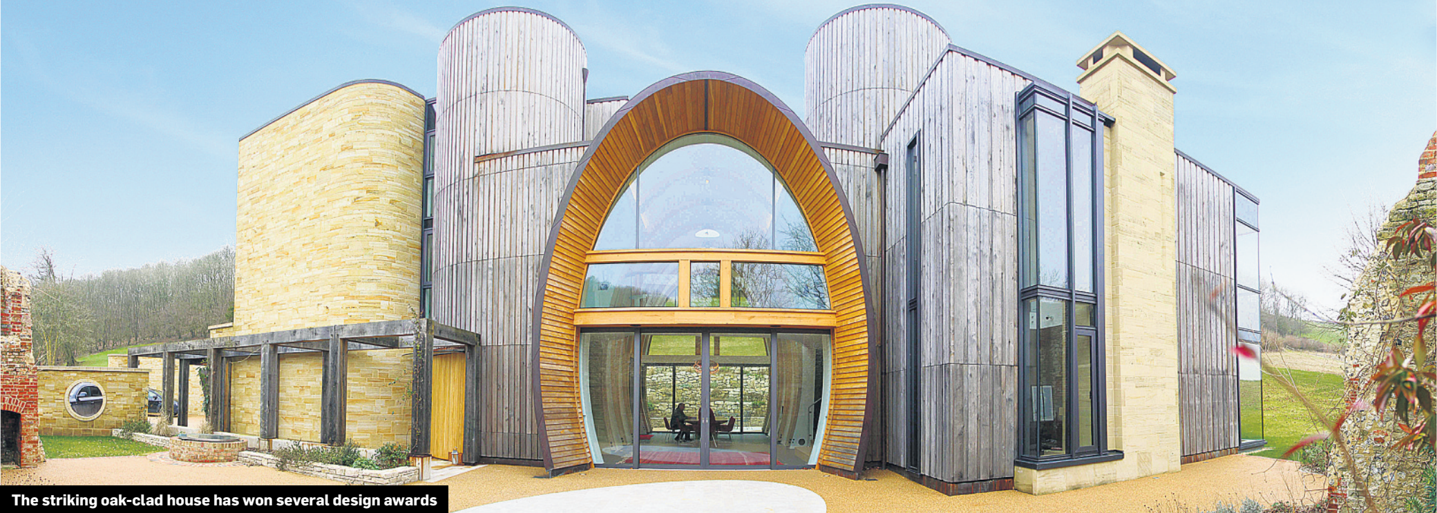
The striking oak-clad house has won several design awards
